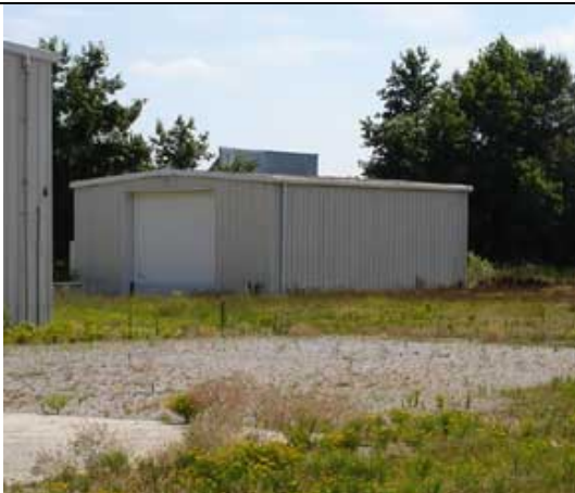
View of Front of 1200 SF Storage Building
